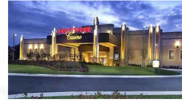
Hollywood (Perryville) (Opened 9/17/2010)
